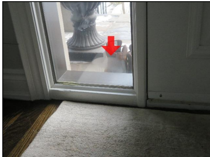
Lost seal on double or triple glazing
