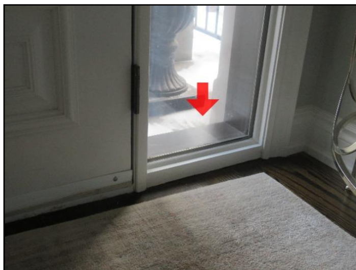
Lost seal on double or triple glazing
