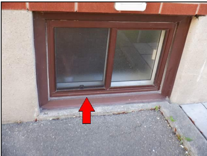
Example: Sealant around windows and doors...
