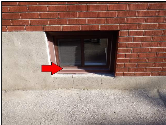
Example: Sealant around windows and doors...
