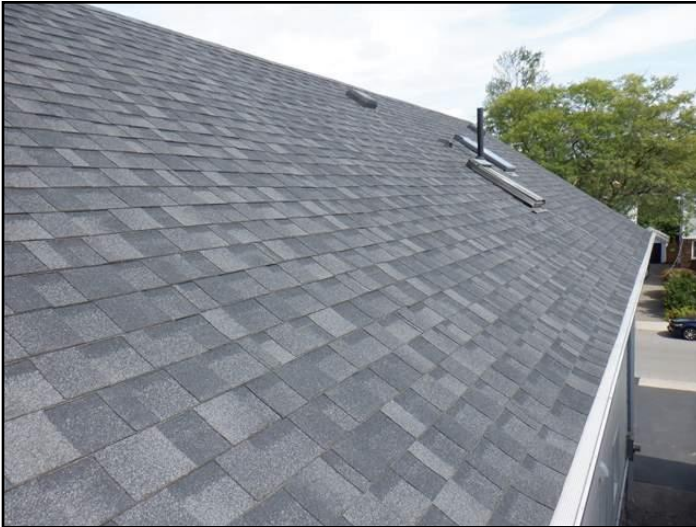
Asphalt shingles
