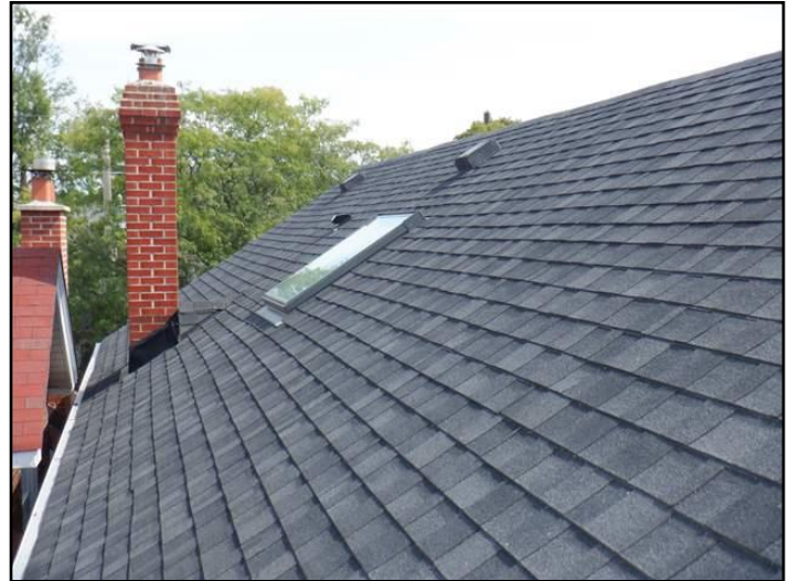
Asphalt shingles
