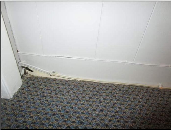
Exposed on walls
