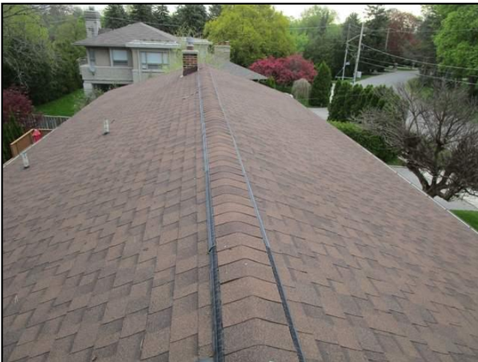
Roof coverings wear out and are replaced...
