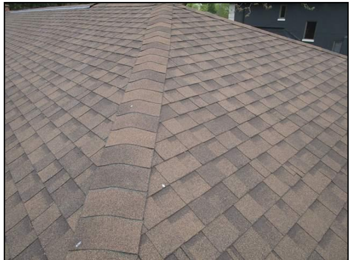
Roof coverings wear out and are replaced...
