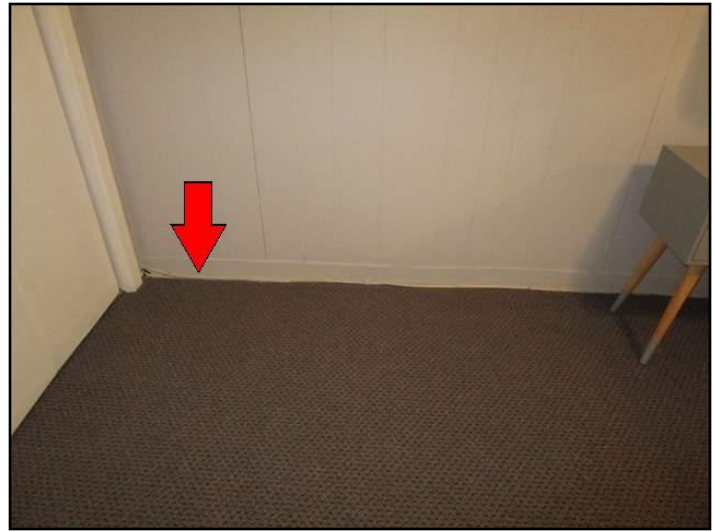
Exposed on walls
