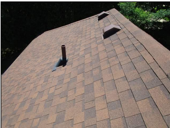
Roof coverings wear out and are replaced...
