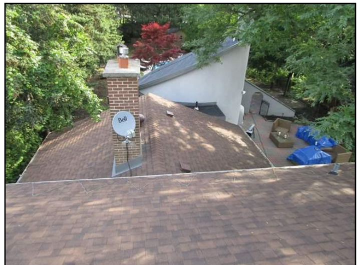
Roof coverings wear out and are replaced...
