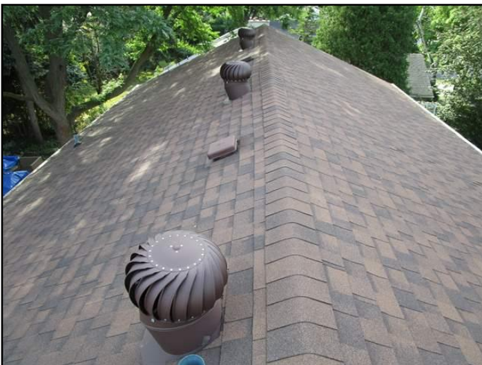
Roof coverings wear out and are replaced...
