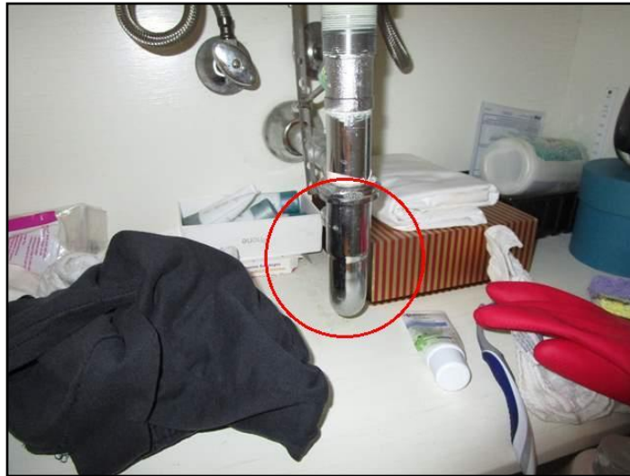
'P'-trap corroded
