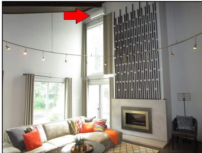
Fan working at indoor unit but not cooling
